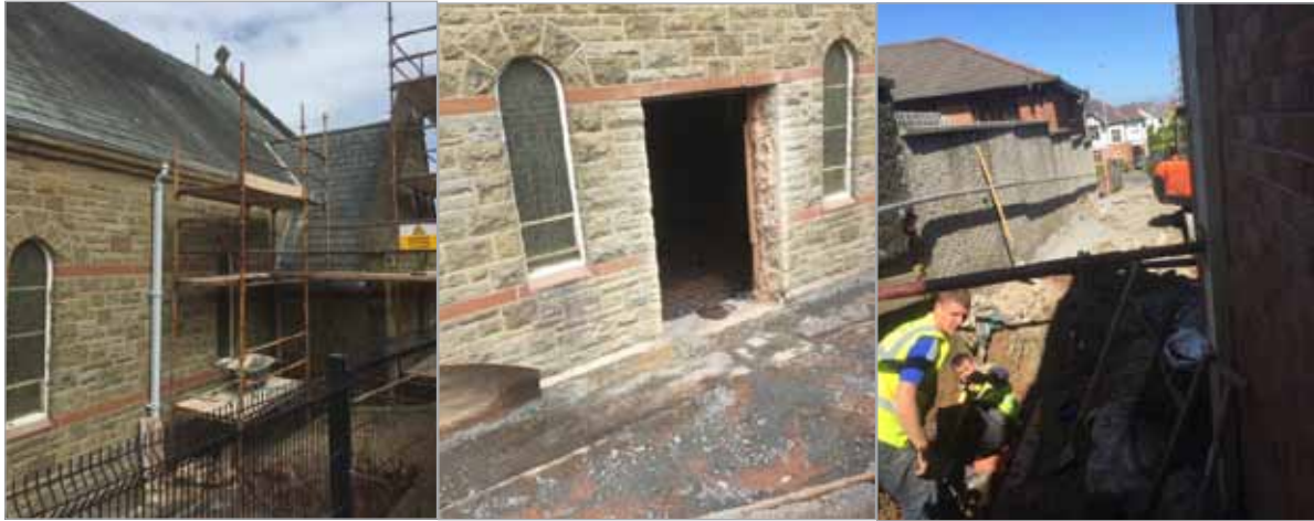
Formation of new doorway into Church & Excavation works for re-routing cables
