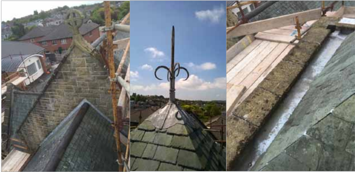
Views from Scaffolding
