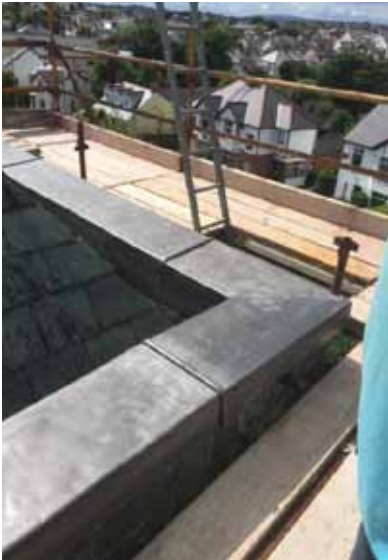
View of Tower
