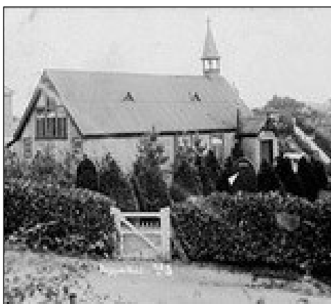
Left Old temporary iron Church, St Mark's Biggin Hill.
