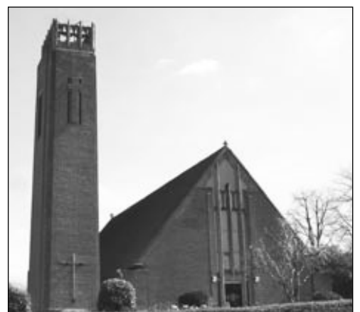
Right New Church built from dismantled materials from All Saints' North Peckham, London.
