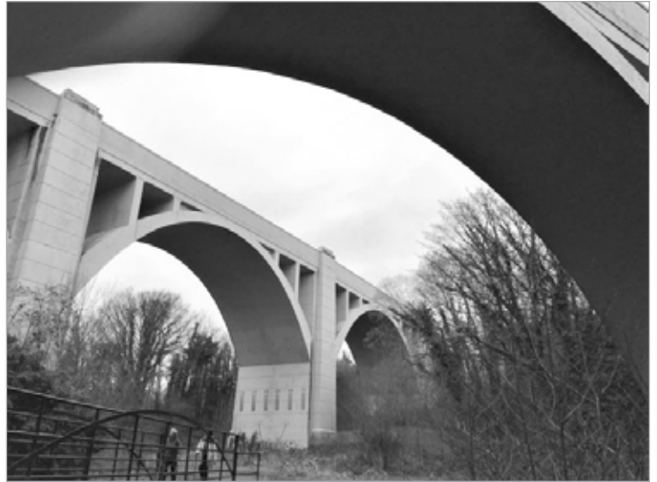
Bleach Green Railway Viaducts
