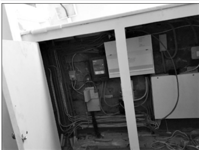
Work on New Fuse Box
