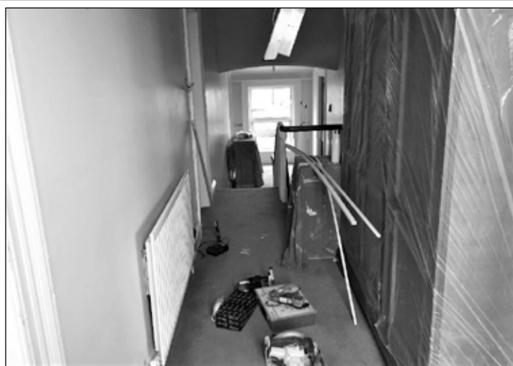
Ongoing Electrical Work
